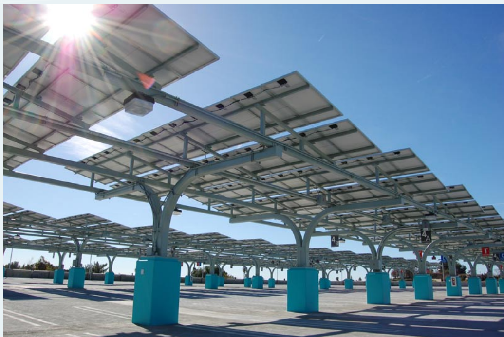
Solar (photovoltaic) panels are installed on a shade structure above a parking structure, Los Angeles Community College District—121 kW—67% electricity offset.
