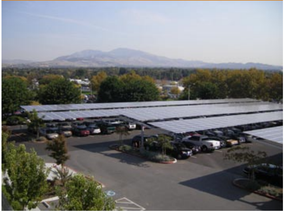
Diablo Valley College in Pleasant Hill, CA has installed photovoltaic panels on shade structures over parking area.
